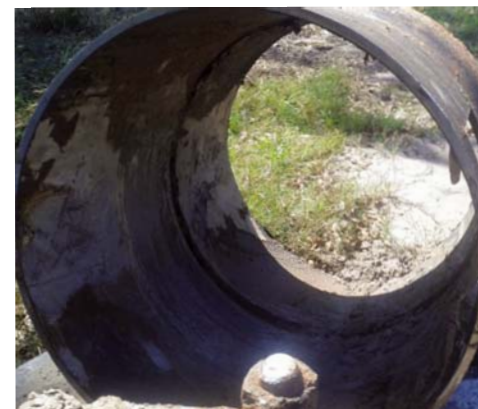
Figure 7. Section of Removed Pipe
