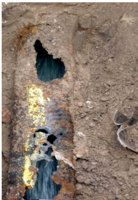
Figure 1. Ductile Iron Pipe Corrosion
